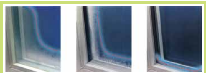
Full Metal Spacer With conventional metal spacers, condensation is a fact of life
